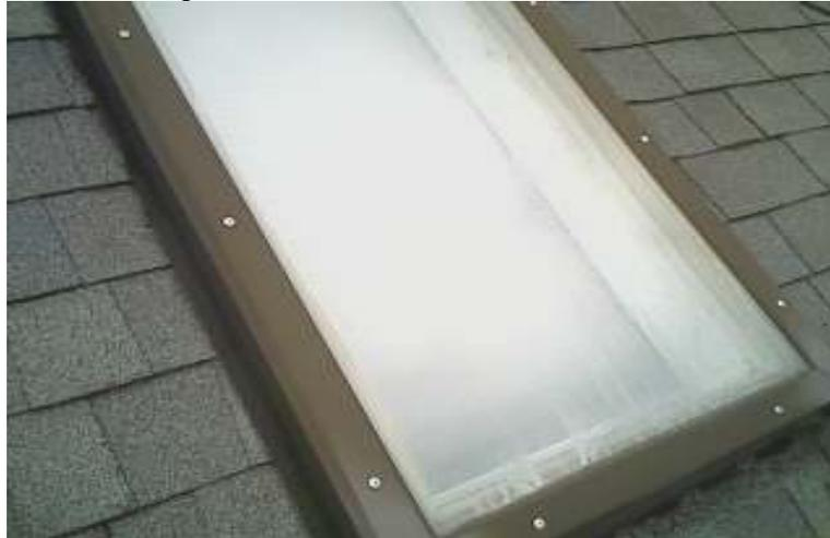
**Water stains** --- Water stains were noted. Stains are evidence of past or present water penetration. Have the source evaluated and repaired or confirmed repaired by a contractor.
