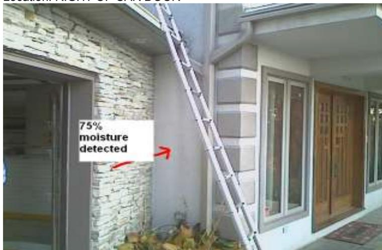
**No isolation gap** --- An isolation gap is a separation of the EIFS between all wall penetrations and expansion joints. This gap allows for placement of a foam backer rod and caulk. This detail is important to help prevent a seal failure. Have evaluated by an EIFS specialist.
