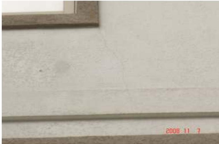
**E.I.F.S below grade** --- The EIFS siding is contact or below grade and is subject to "wicking", this condition should be further evaluated by an approved EIFS specialist and corrected prior to close.
