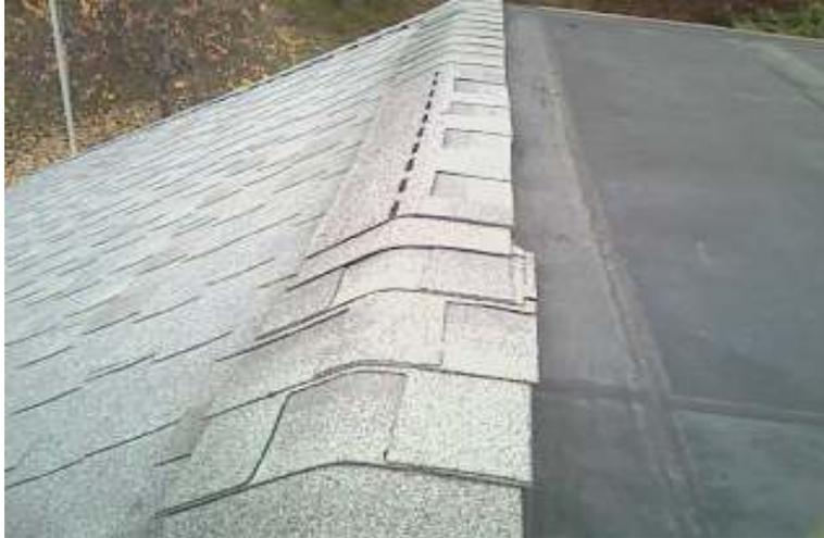
**Missing/cracked shingle** --- Roof has missing or cracked shingles that should be repaired by a qualified roofing contractor. Water penetration could occur at these areas. Have the contractor further evaluate the roofing system for repairs.
