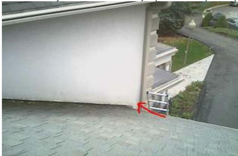
**Elevated moisture** --- There were elevated moisture readings at the below noted location. Elevated readings could indicate an active moisture concern or raise the likelihood of mold, mildew, and/or dry rot. Determine the source of the moisture and correct.
